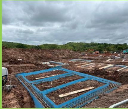
The Hem – on site - Vistry – completion date – Apr 29
