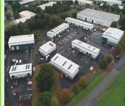
Hortonwood Plot 12 – TWC – Operational
