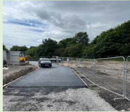
Pool Hill Road Site D – in progress
