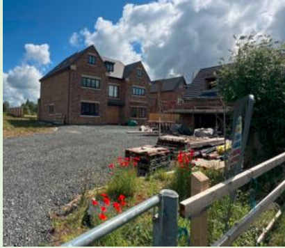
Horton Lane Plot A1 – on site – Private purchaser – completion date - Oct 24
